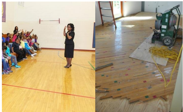
Gymnasium flooring from the former Campostella Elementary School in Norfolk (left) was salvaged and repurposed in the Brock Environmental Center (right).
