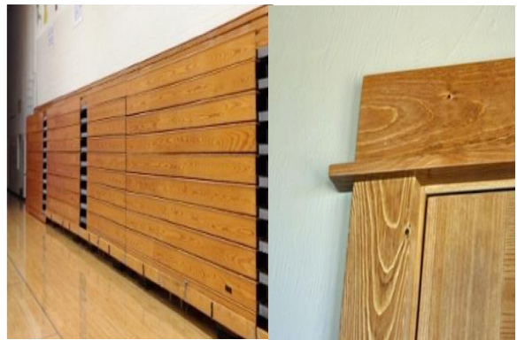
Bleachers from Virginia Beach's Salem Middle School (left) were reused as trim for doors and windows in CBF's Brock Environmental Center (right).
