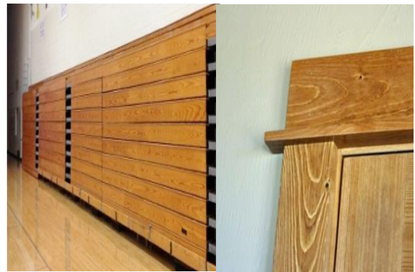
Bleachers from Virginia Beach's Salem Middle School (left) were reused as trim for doors and windows in CBF's Brock Environmental Center (right).
