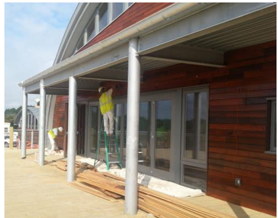
CBF used "sinker cypress" (cypress logs that have been drowned in rivers for years) like the one pictured above as exterior wall finish at the Brock Environmental Center (pictured below).
