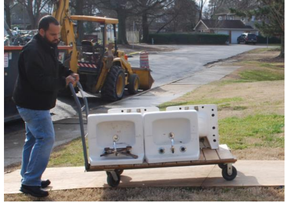
Sinks from the former Lake Taylor Health Center in Norfolk have been reused in the Brock Environmental Center.
