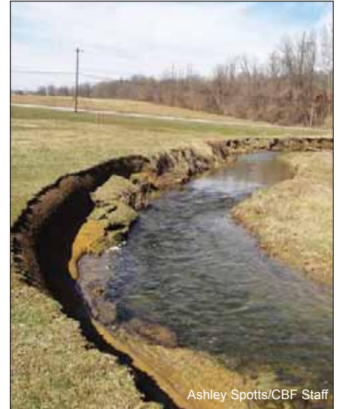
The East Branch of the Octoraro needed various improvements.
