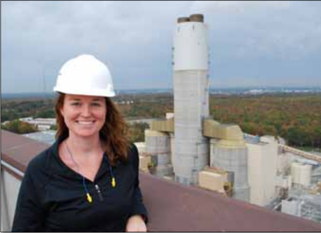
In response to a 2006 Maryland air pollution control law, Constellation Energy built this scrubber at its Brandon Shores coal-fired power plant and hired 32 workers in part to run and monitor the scrubber. Among those hired was chemical technician Melissa Sampson (above).
