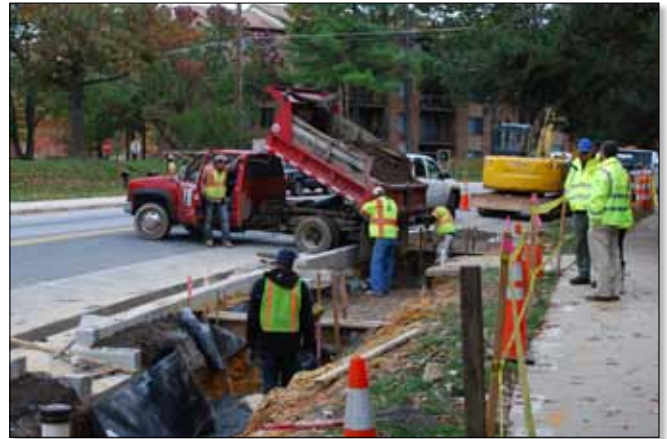
Construction workers in Montgomery County, Maryland, build stormwater control devices that look like roadside gardens.
