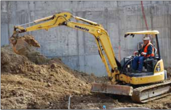
Construction crews are working to improve sewage treatment plants across the Chesapeake Bay region.
