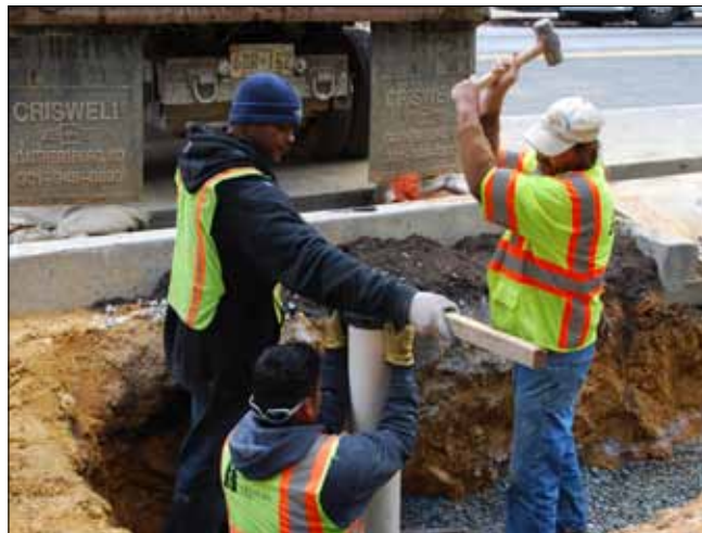
Workers build a stormwater pollution control device called a “bumpout” in Montgomery County, Maryland.
