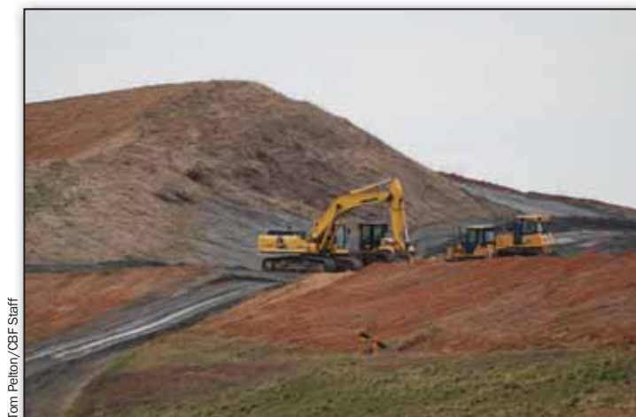
Fly ash is waste that is produced by the burning of coal and captured in power plant pollution-control systems, before being landfilled.
