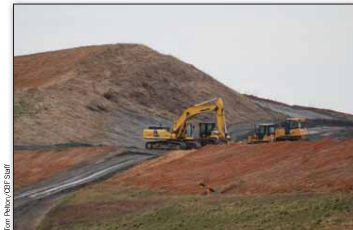
Fly ash is waste that is produced by the burning of coal and captured in power plant pollution-control systems, before being landfilled.
