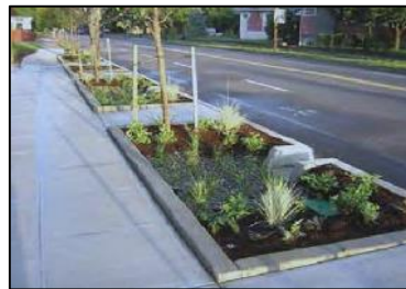
Figure 3: Examples of road-associated “green” stormwater management
