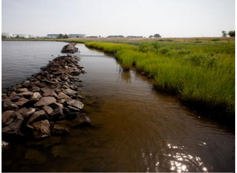
The rocky shoal and ten-foot berm help reduce flooding and erosion from storm surges and wave action from the Elizabeth River.
