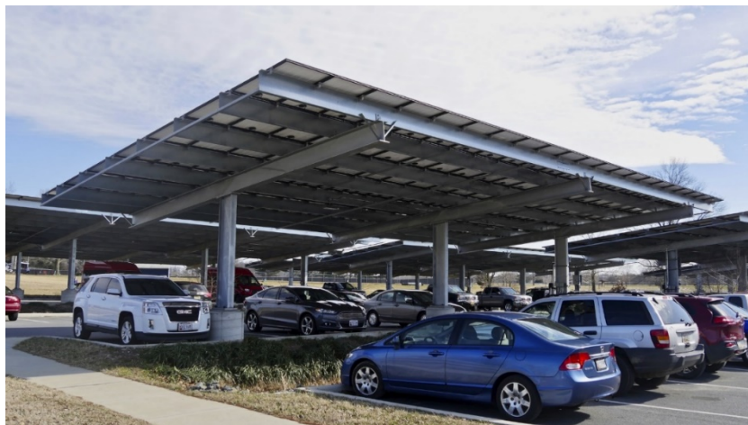
Chesapeake College, Wye Mills, Maryland
