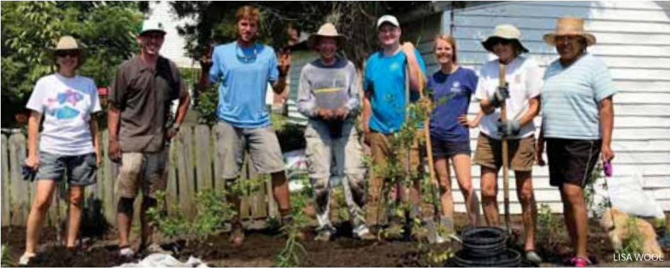
Volunteers helped install 10 projects throughout Cambridge to slow and filter polluted runoff before it hits local waterways.
