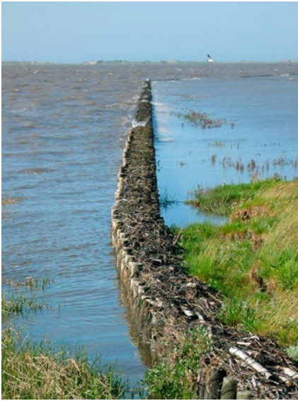
Example of Brushwood groyne (Eden and Thorenz, 2024)
